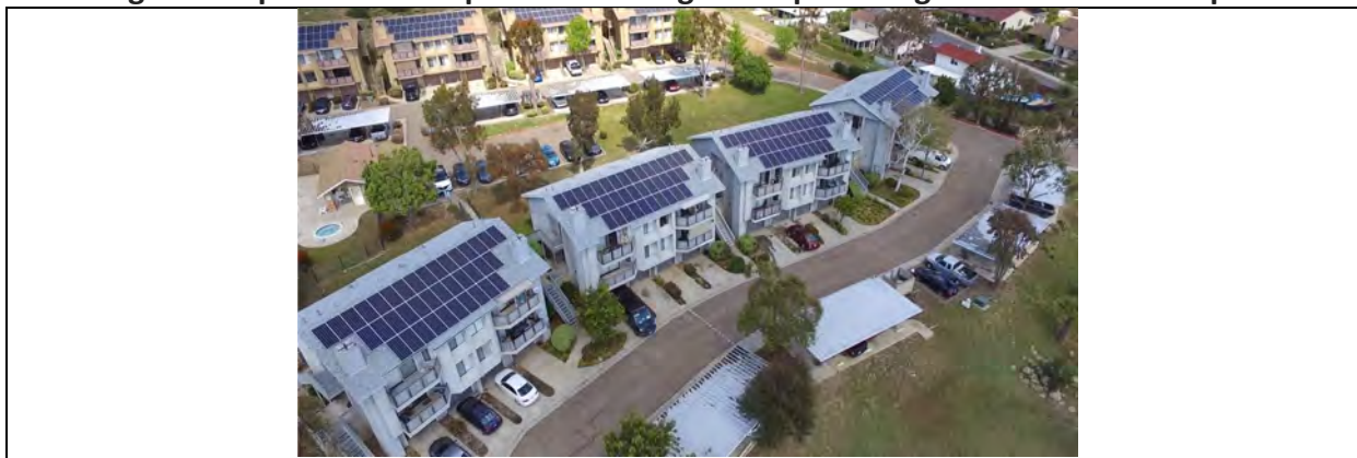
Figure 7. Apartment complex in San Diego area providing tenants with solar power
