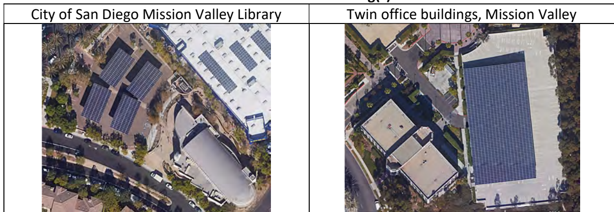
Figure 4. San Diego examples of parking lot solar exceeding roof area of associated commercial building(s)
