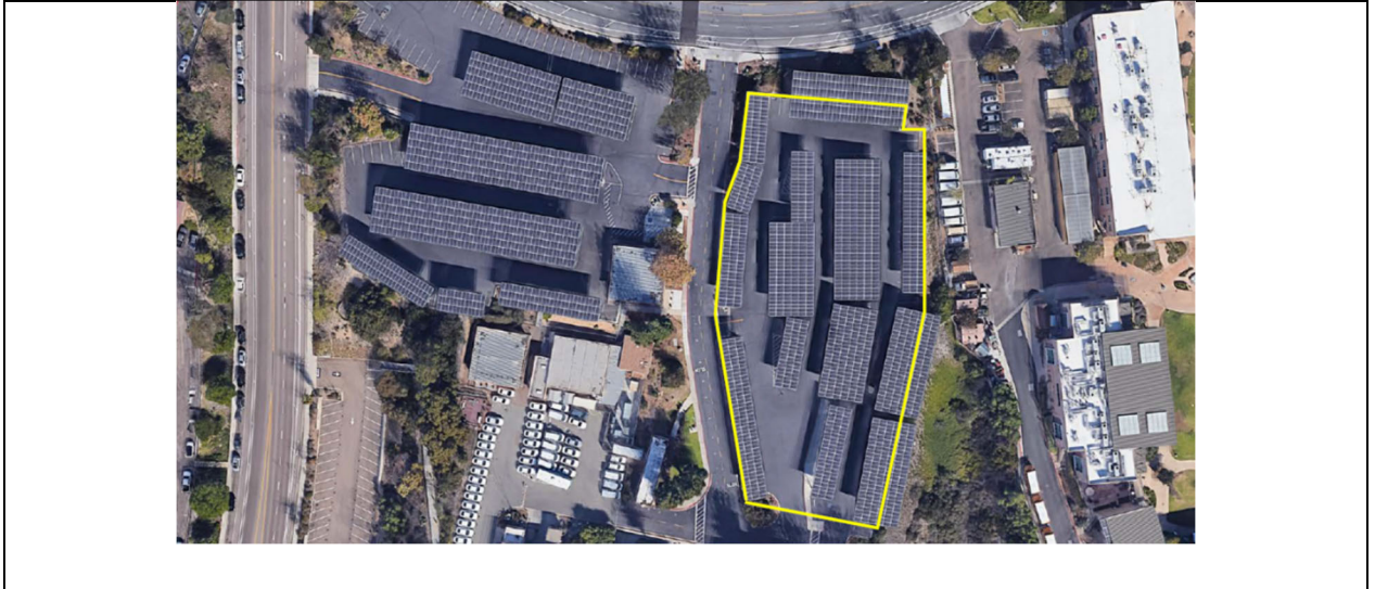
1 Figure 1. San Diego County Office of Education Park Lot Solar Arrays 18
